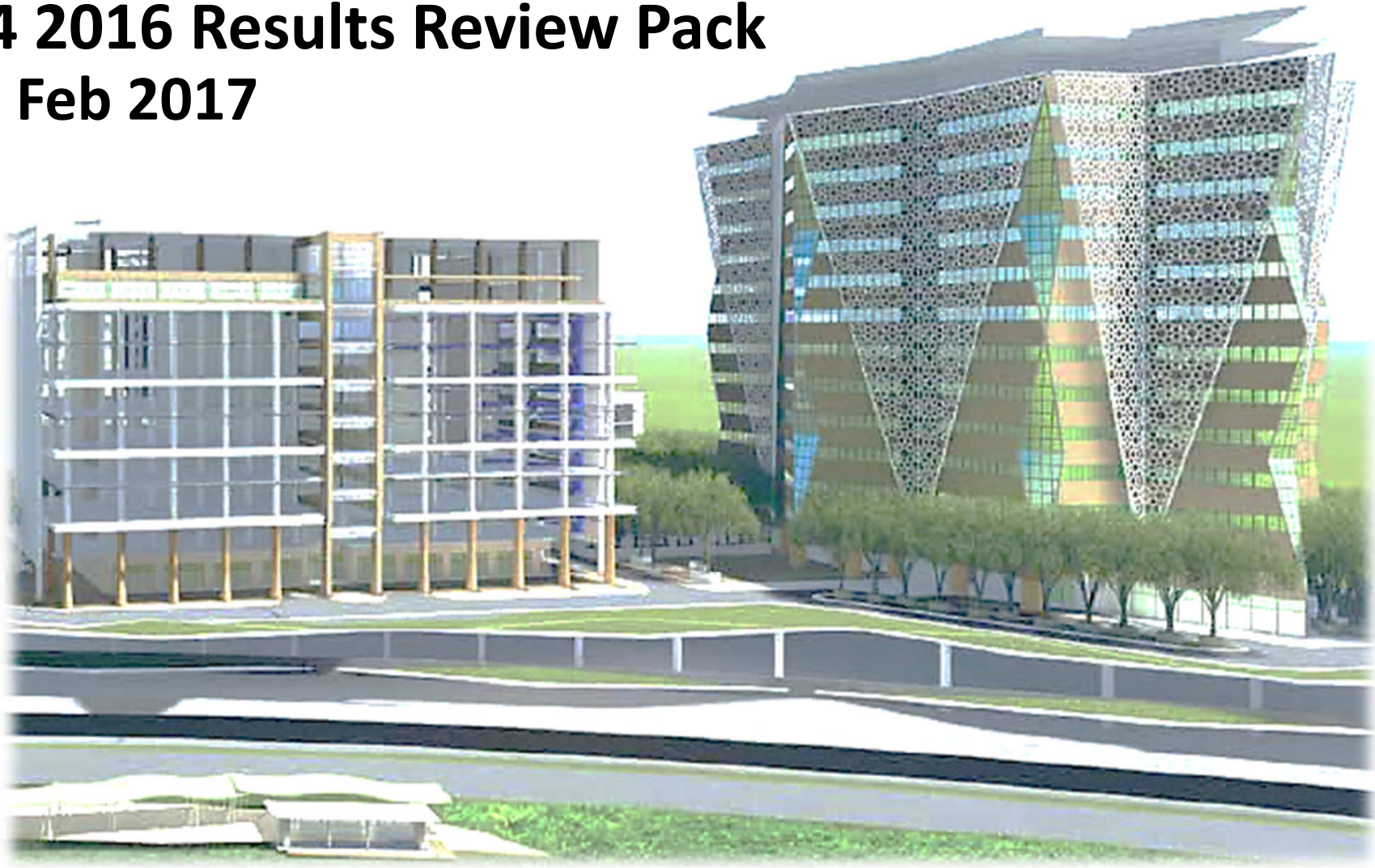
Picture illustrates the use of VDC in our Parcel F, Putrajaya project
